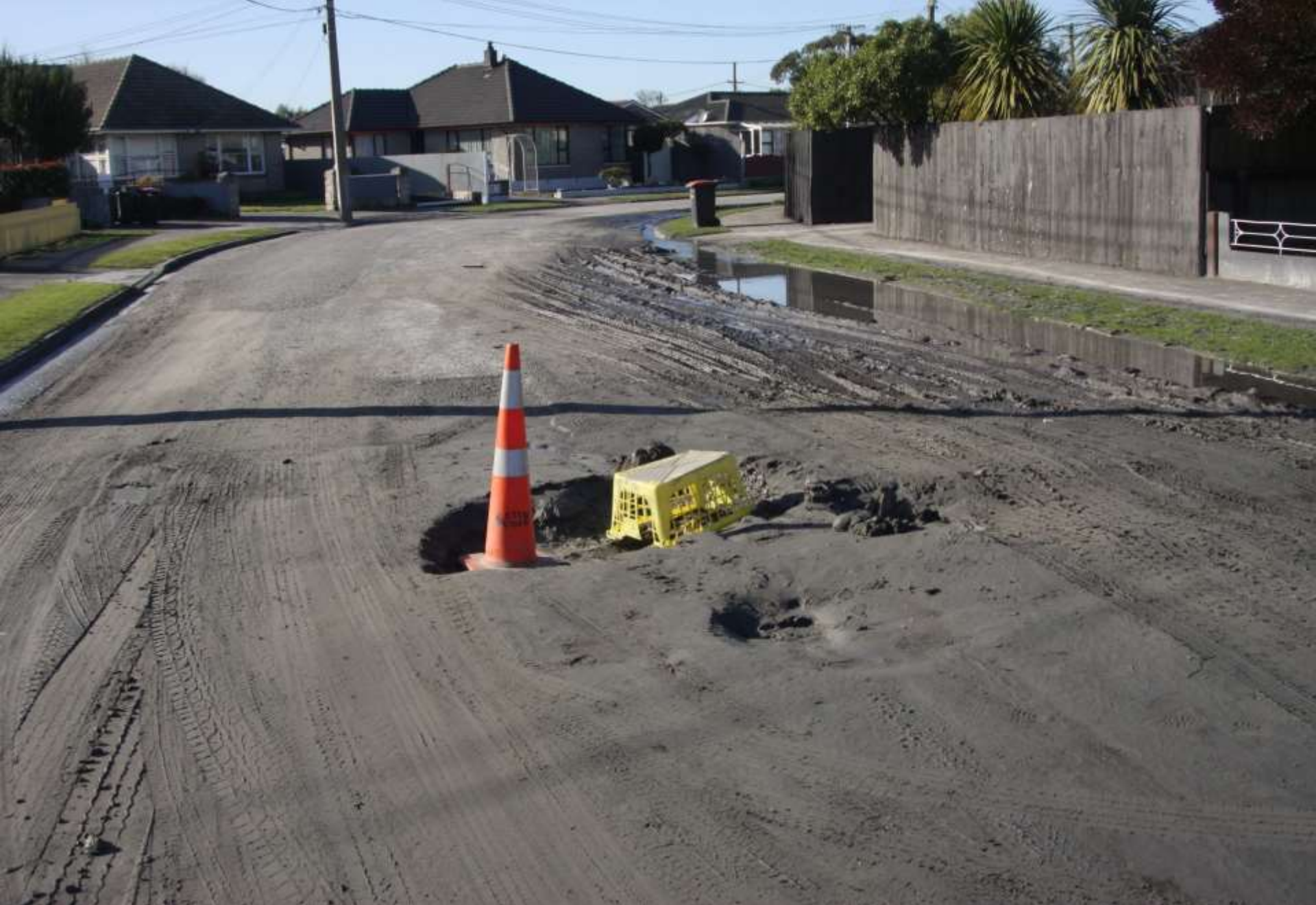
Liquefaction – Christchurch East, June 2011
