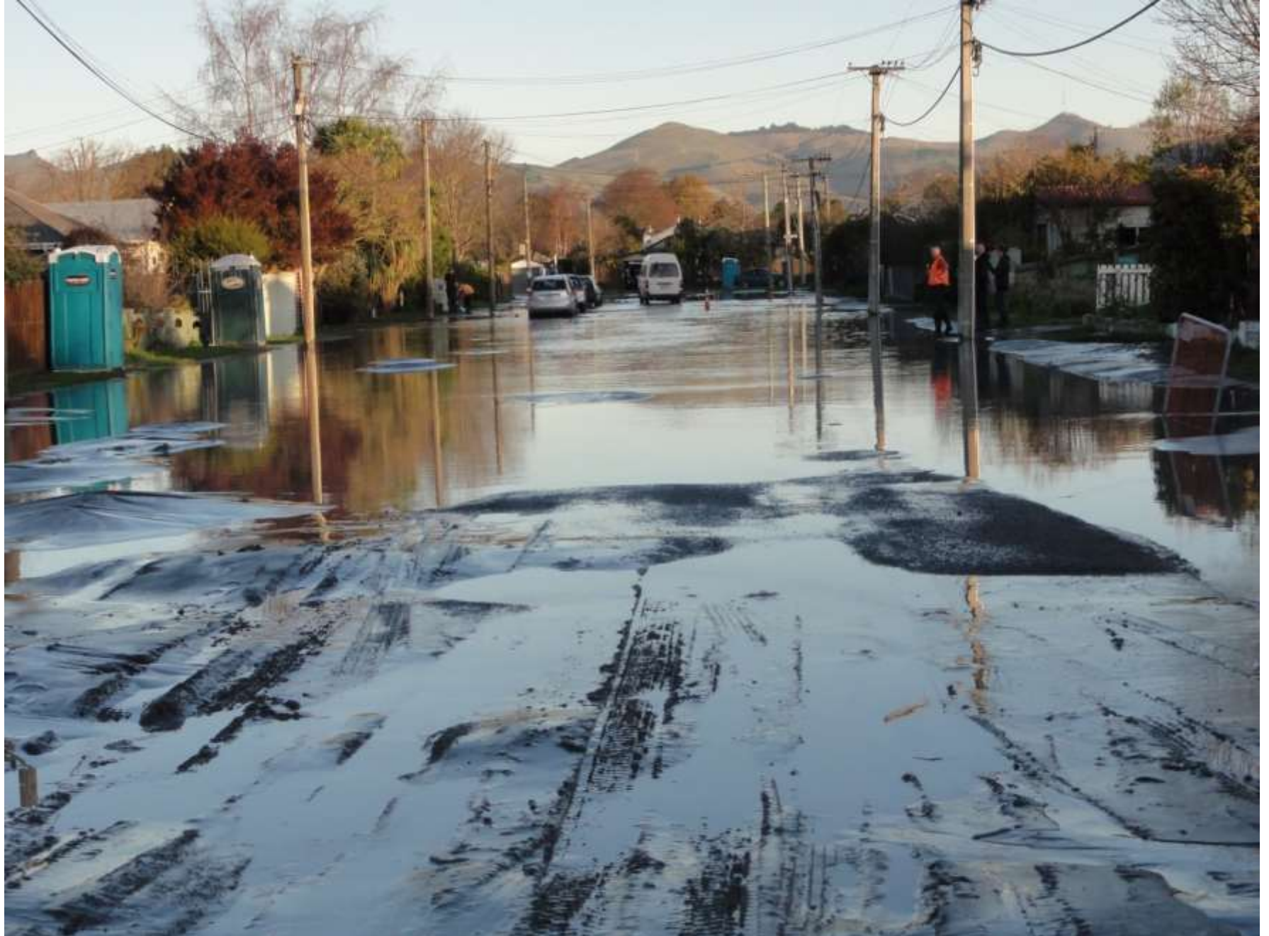
Liquefaction – Christchurch East, June 2011 (Courtesy Merrick Taylor)
