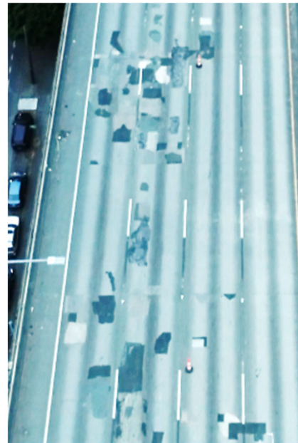
I-5 Ship Canal Bridge Deck Rehab
